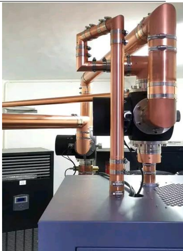
Fig. 3. Assembly of the feeding and balanced-to-unbalanced transition components. Source: Authors' field photograph
